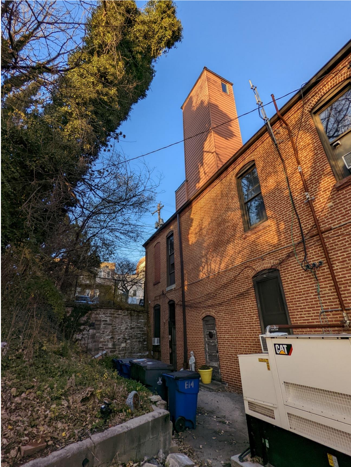
Image 8: West elevation at the rear of the property. The rear two bays of this elevation are a 1902 addition. Also visible is the stone retaining wall, which demonstrates the significant grade change between Booth Street, an alley street, and Hollins Street.
