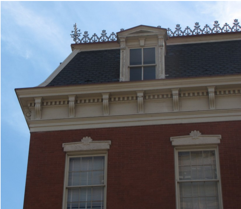
Detail photo of cornice, mansard roof, dormers, and roof cresting.
