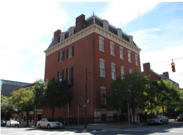
View of the north façade and east elevation.
