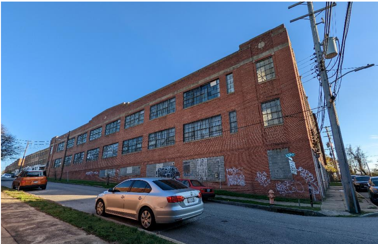
Image 16: North elevation, facing 32 nd Street.
