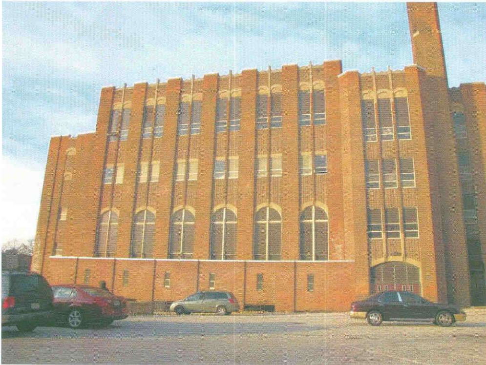
The auditorium wing offers an excellent view of the window and roof details (view from south).
