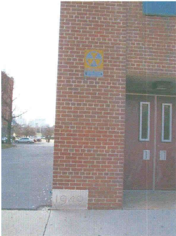
Cornerstone for the South Addition on Caroline Street.
