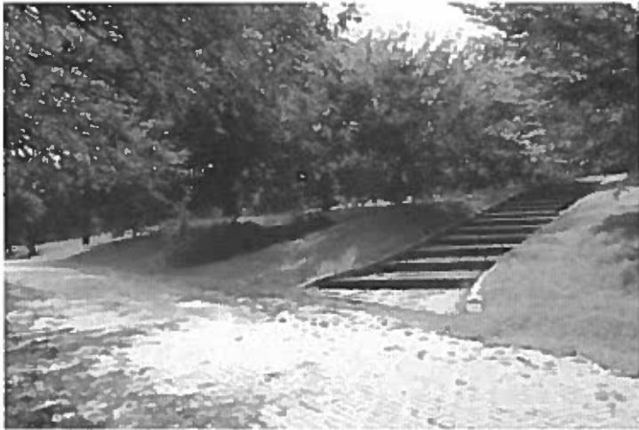
Image 7 – Historic Path, stairs, and stone wall
