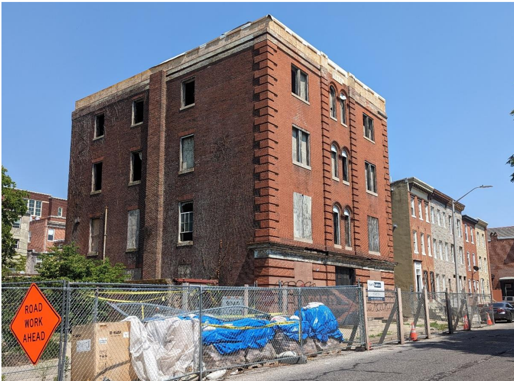
Image 20: Façade and west elevation.
