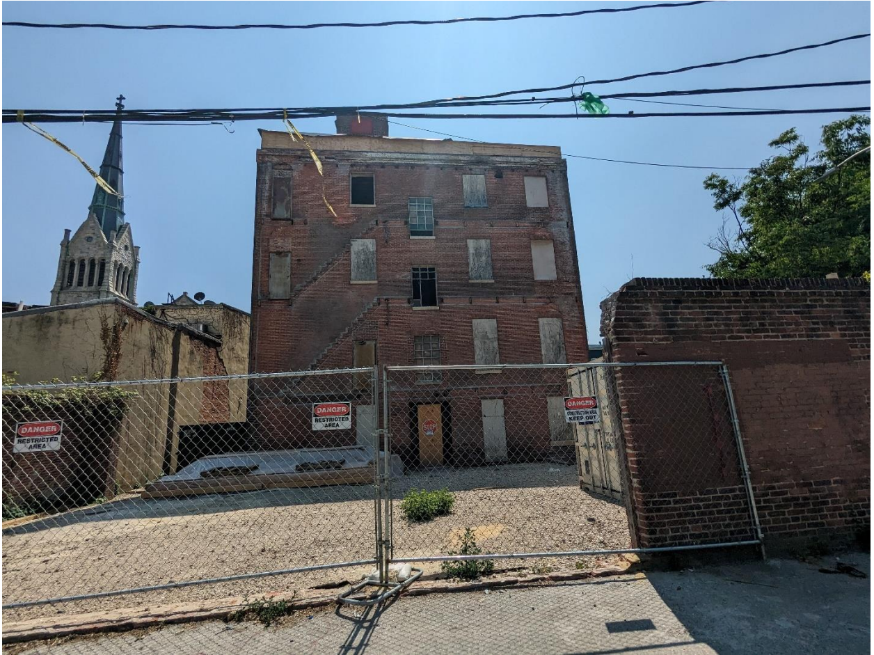
Image 22: Rear elevation, viewed from Stoddard Alley.
