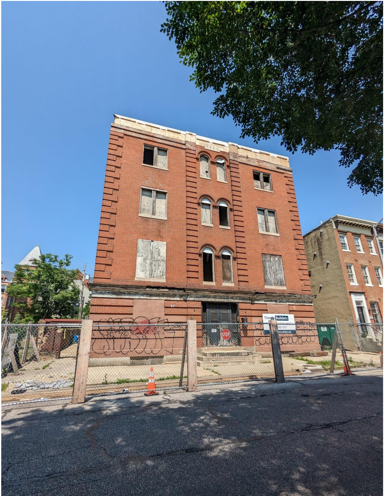
Image 18: Façade, facing Druid Hill Ave.
