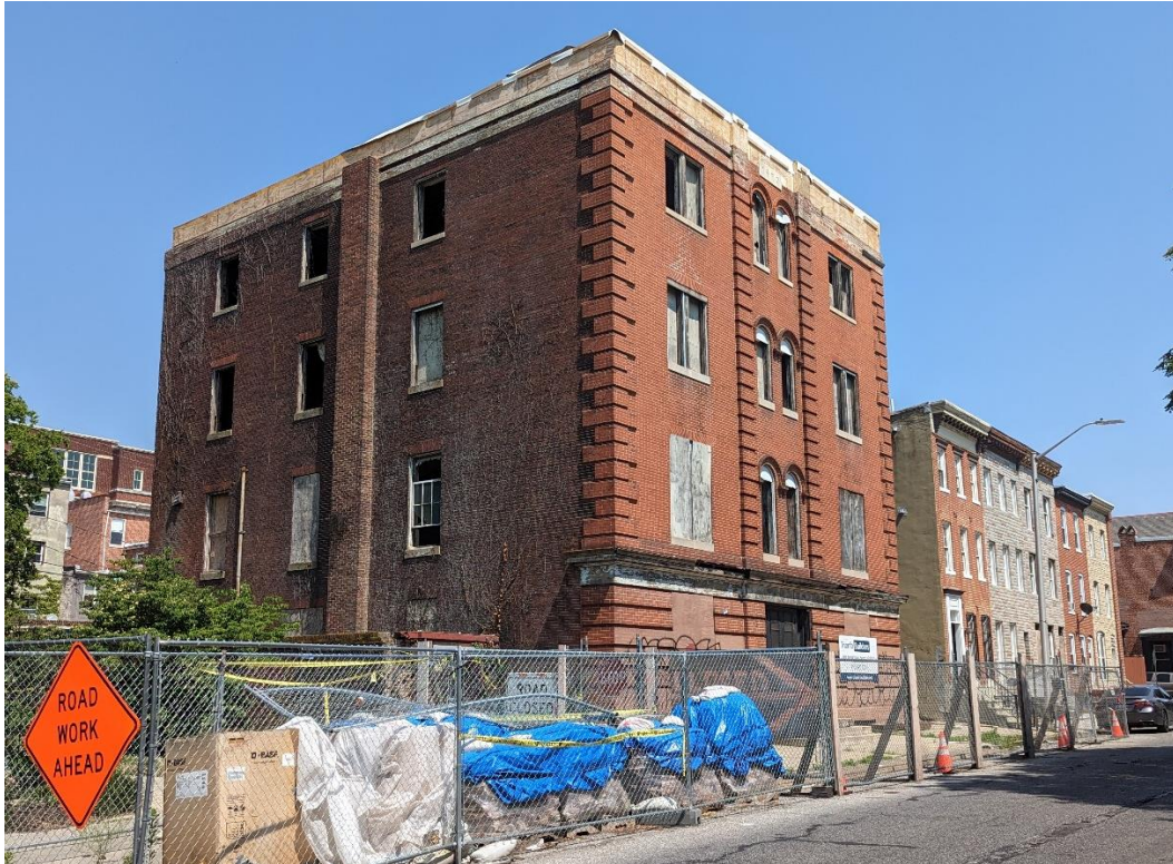
Image 20: Façade and west elevation.
