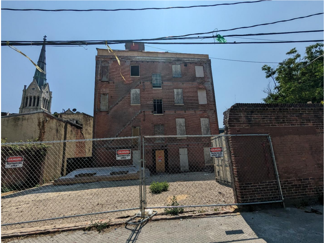
Image 22: Rear elevation, viewed from Stoddard Alley.
