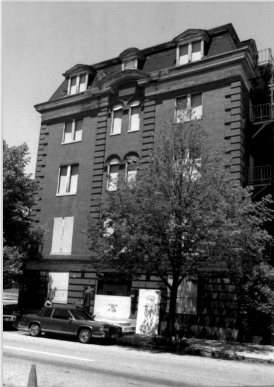
Image 15: The façade of the Home of the Friendless in June 2002 (Fred B. Shoken, “Home of the Friendless” National Register of Historic Places Nomination Form (Washington, DC: U.S. Department of the Interior, National Park Service, 2002))
