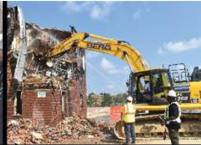
PERKINS HOMES DEMOLITION
