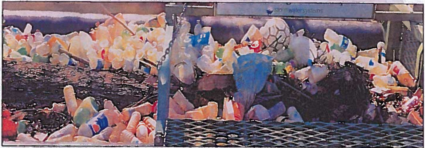
Figure 3 - Close-up of litter caught in the Anacostia Bandalong Trap
