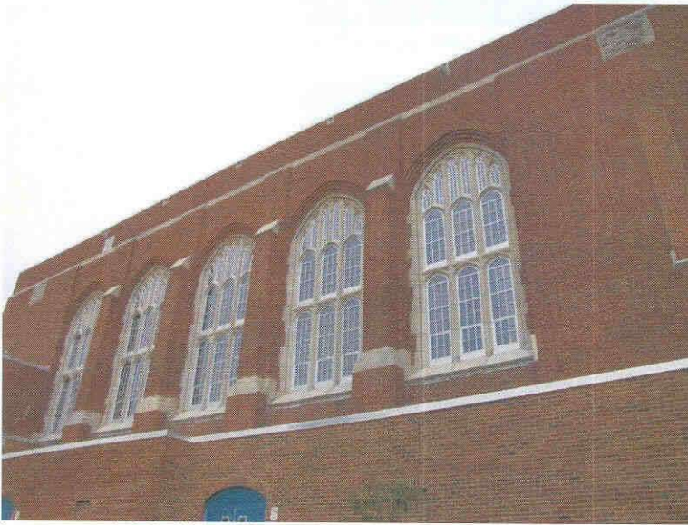
Large traceried Gothic windows.
