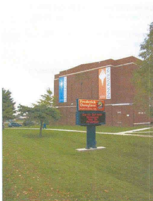
View of the eastern wing from Gwynns Falls Parkway.
