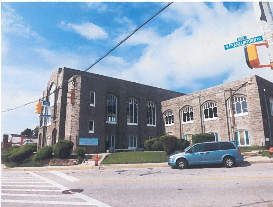
Side elevation viewed from N. Franklinton Rd.
