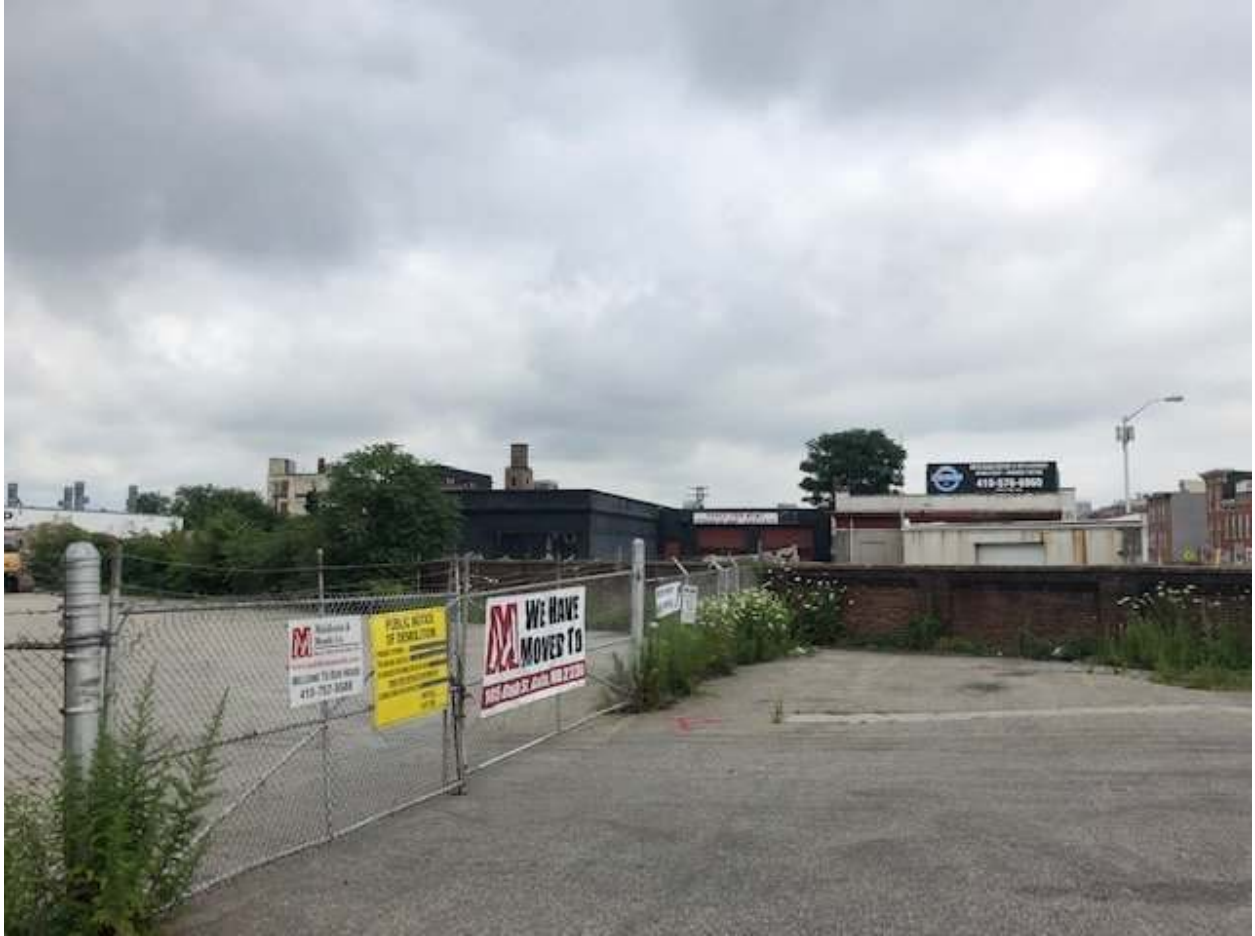
Warehouse on the 1800 block of S. Hanover St.
