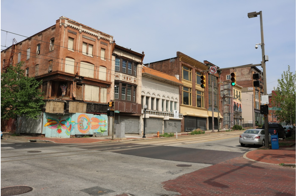
West Side of the 400 Block of North Howard Street
