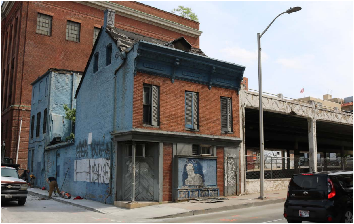
West Mulberry Street facing north into the district
