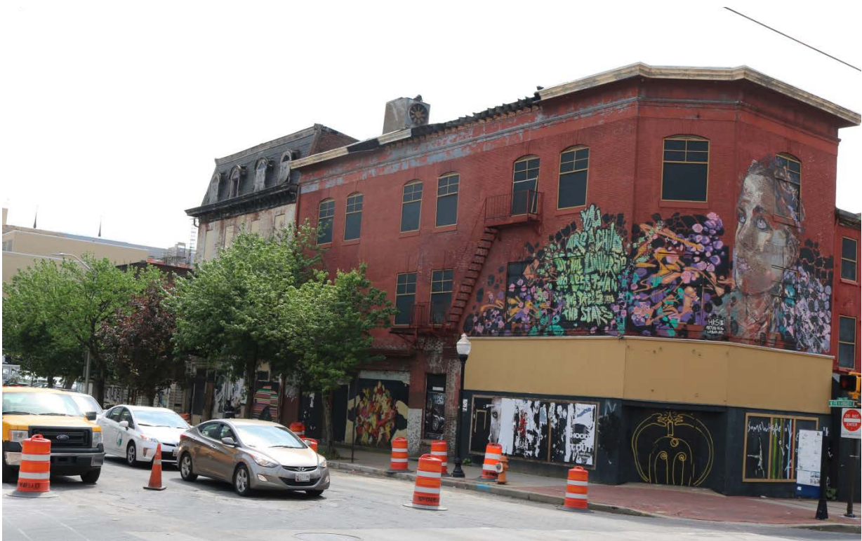
West Franklin Street facing southeast
