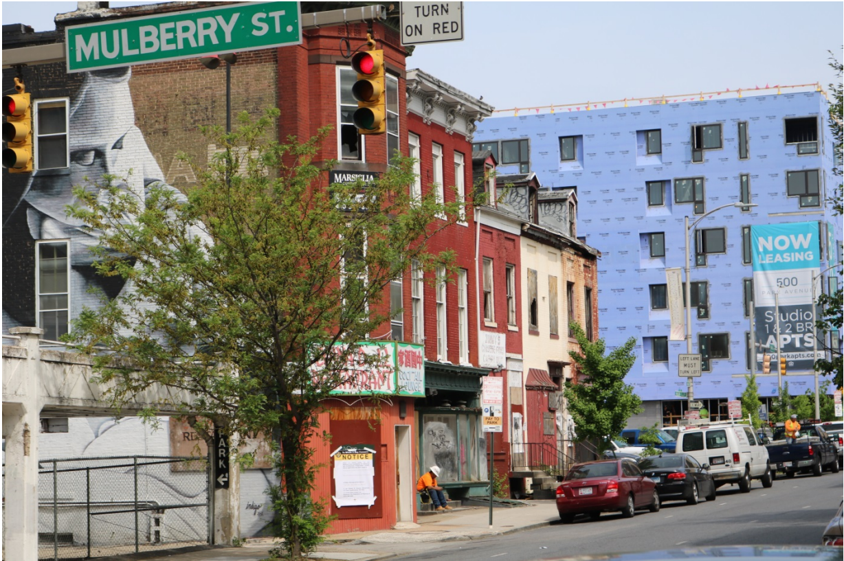
West side of 400 Block of Park Avenue
