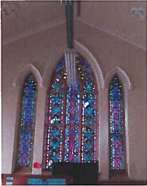
Image 13: Interior view of 1871 church façade windows, facing Carrollton Ave.
