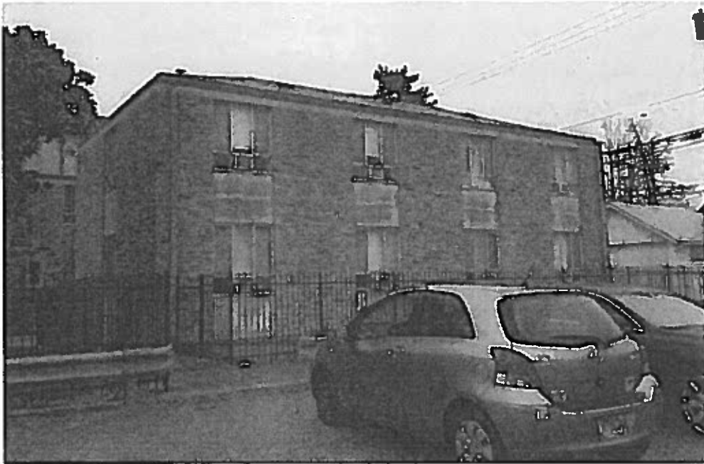
Image 10 – Rear of the 1957 addition.
