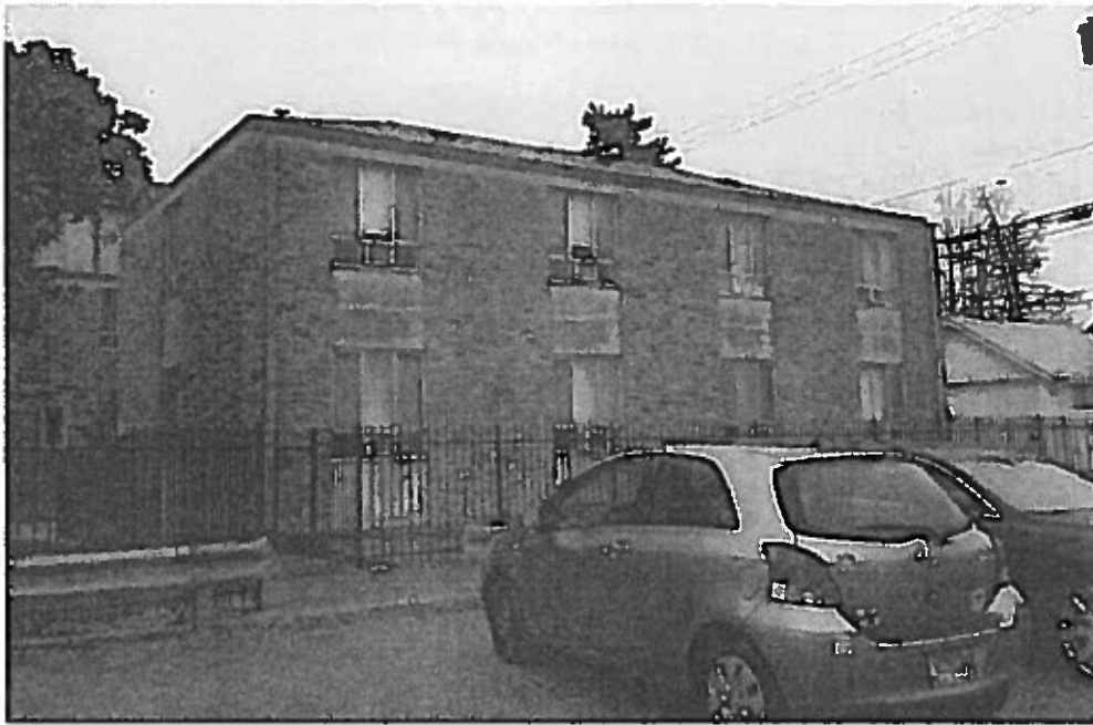
Image 10 – Rear of the 1957 addition.
