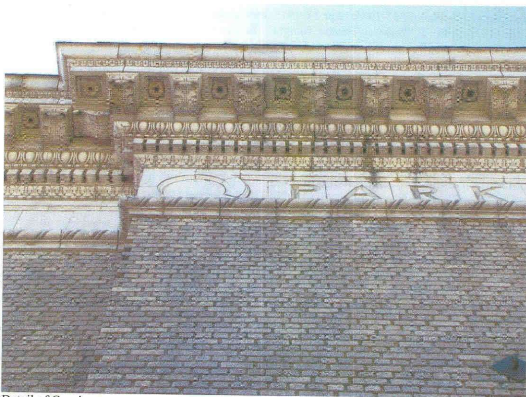
Detail of Cornice.
