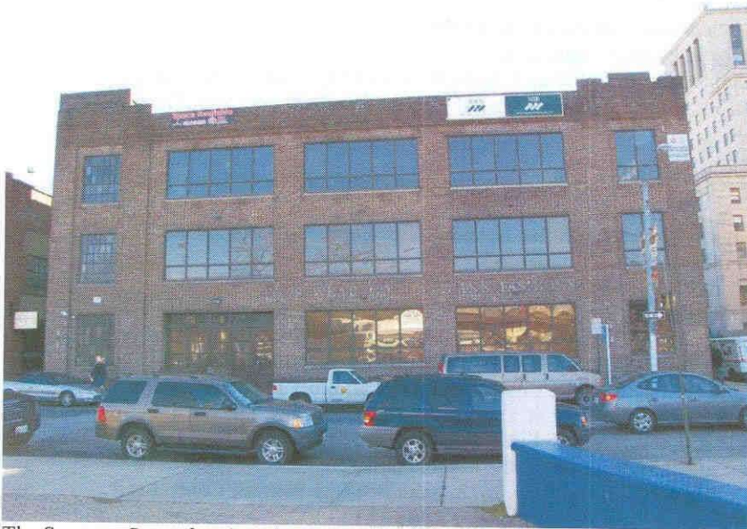
The Saratoga Street façade. Still visible on the building are the remnants for the sign “Diane Fashions” and “Boy’s Wear Co” above the first floor windows.
