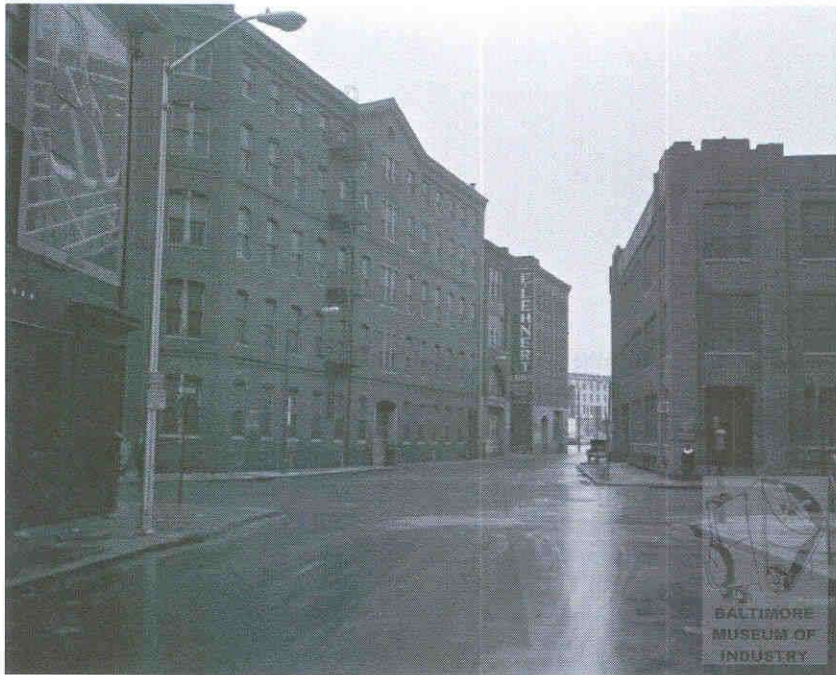
Image 1- View east on E. Saratoga St. of the intersection of Saratoga and Holiday Streets, taken in 1971. The C.J. Youse Building is on the right. (BGE Collection at the Baltimore Museum of Industry.)
