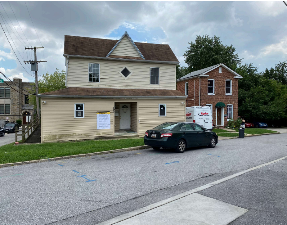
Benninghaus Road Facade
