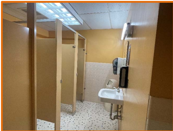
Restroom with original flooring
