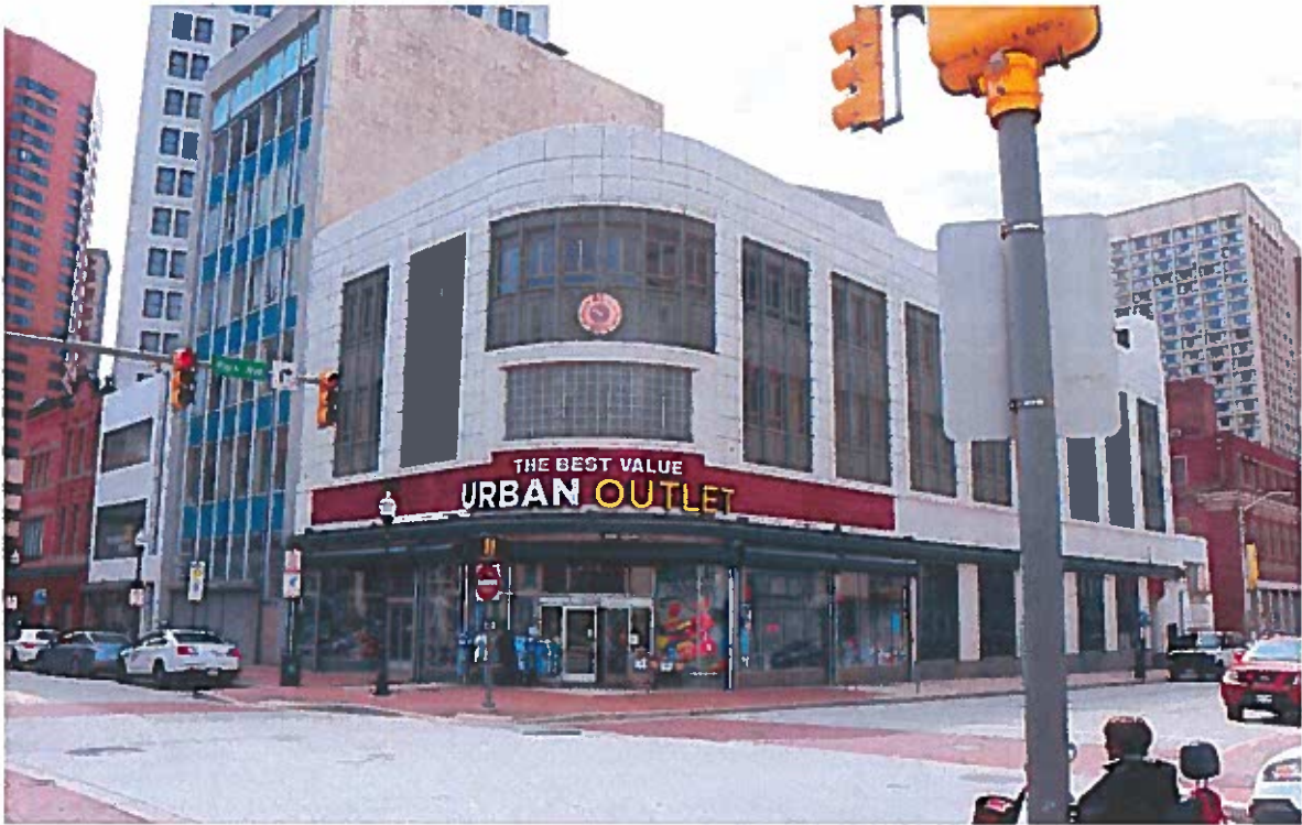
Corner of Park Ave and West Lexington Street facing southeast
