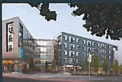
The Fitzgerald 2008 20 Year PILOT 280 Apartments 14,000 SF Retail 1250 Space Parking Garage
