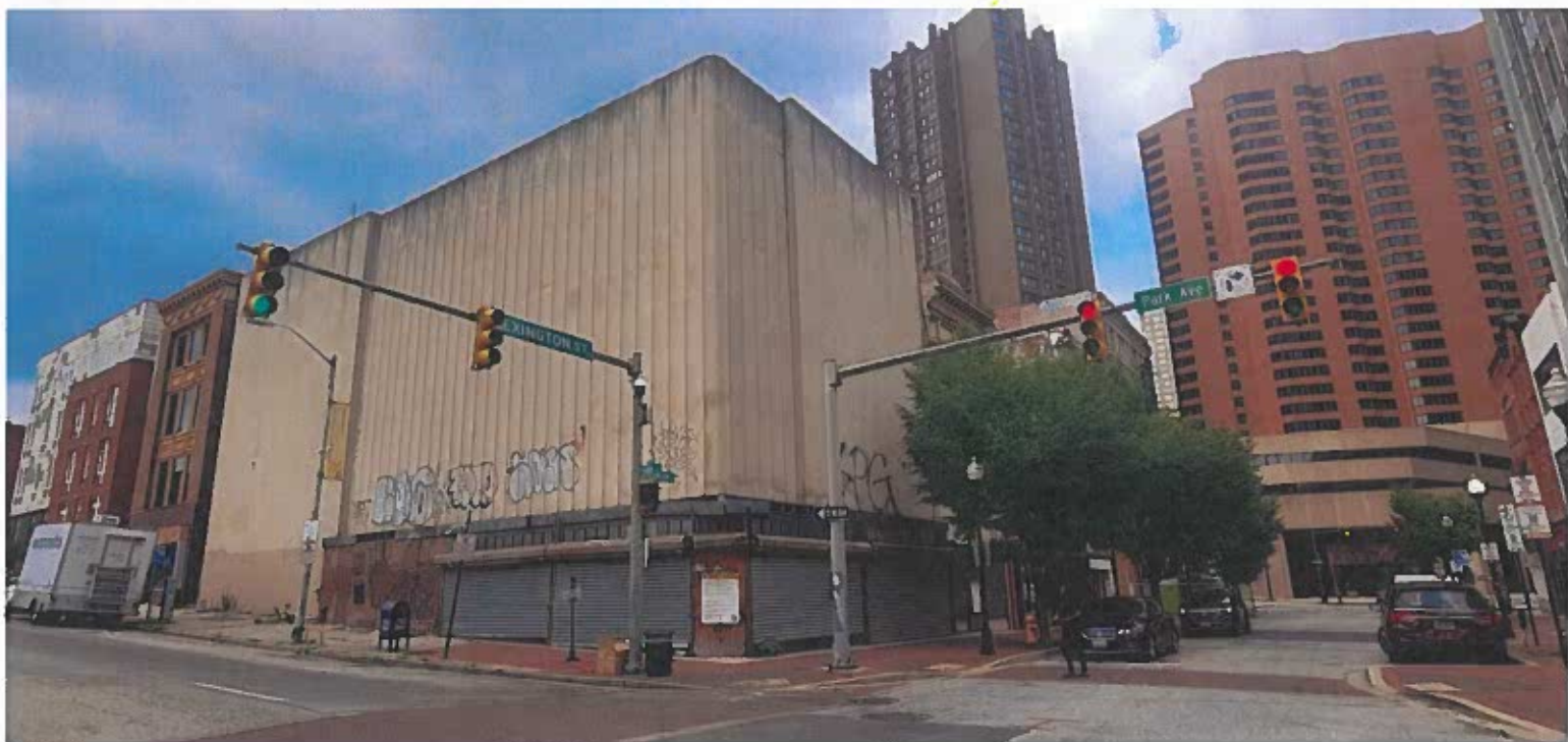
A former Ann Lewis Shops department store at Park Avenue and West Lexington Street. Photo by Ed Gunts.
