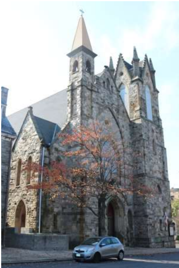
Image 6: View of 1876 church façade on W. Lanvale St.
