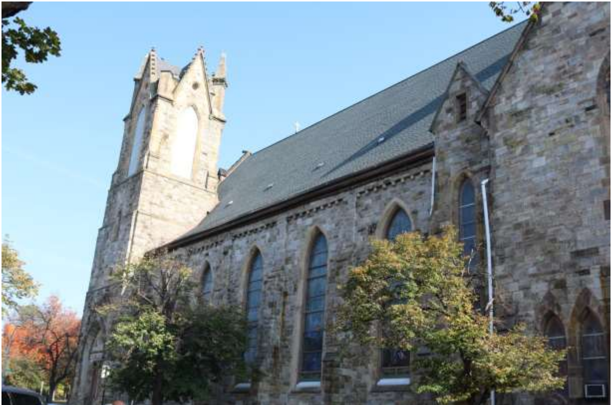
Image 14: View of side of 1876 church (left) and façade of 1871 church (right). Note how seamlessly the structures blend together.
