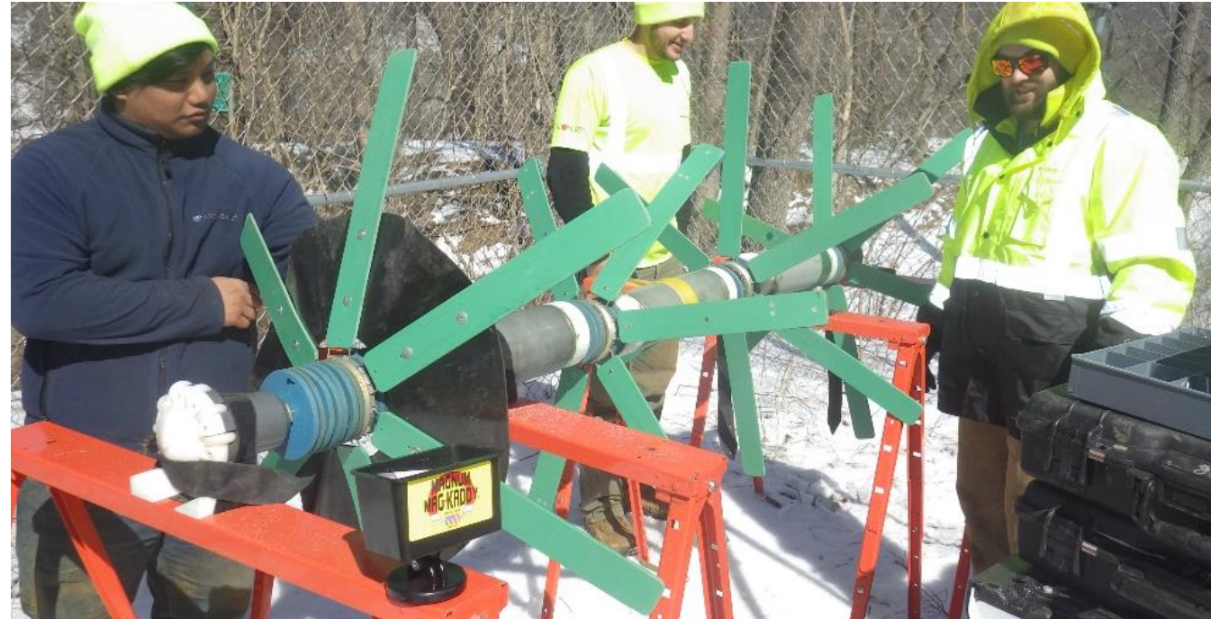
Pipe Diver tool shown for Electromagnetic in-service pipe inspections
