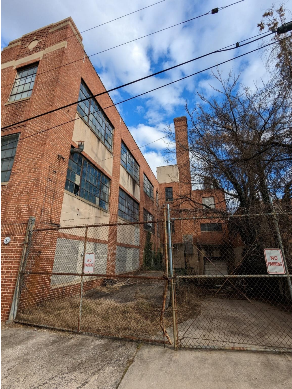
Image 22: The south elevation (left), chimney tower, and loading dock as viewed from Falls Cliff Road.
