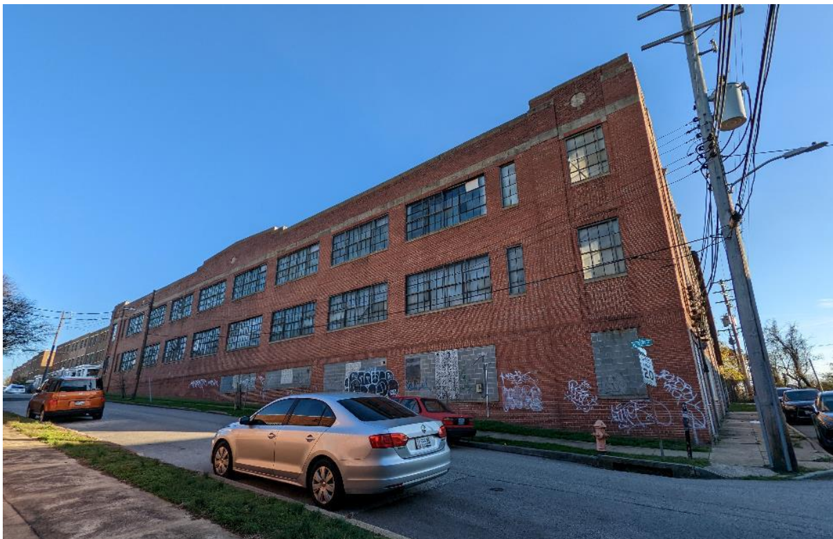
Image 20: North elevation, facing 32 nd Street.
