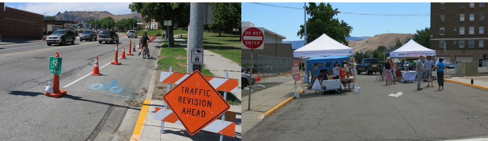
The bike lane added to the westbound portion of Orondo, left, eliminated space that some drivers would use to illegally pass cars in the left travel lane. The half block of Methow that was closed, right, provided space for the pop-up community events during the project, in addition to removing another conflict point from the complex intersection.
