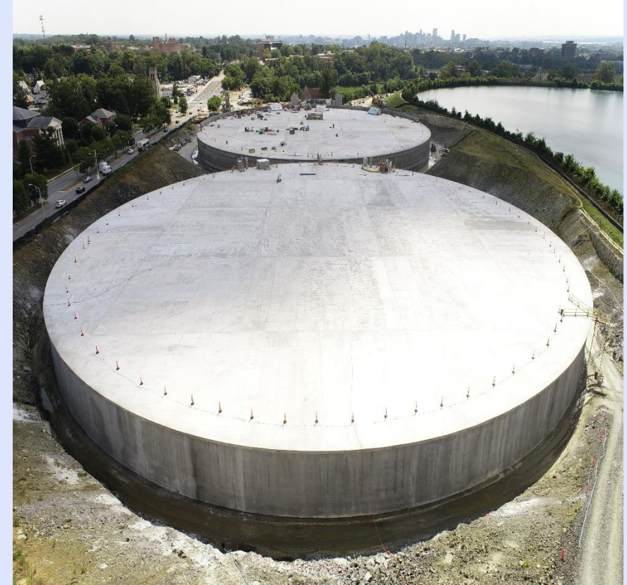
Tank A & B roof and wall pours completed (aerial view) – 8/26/2022
