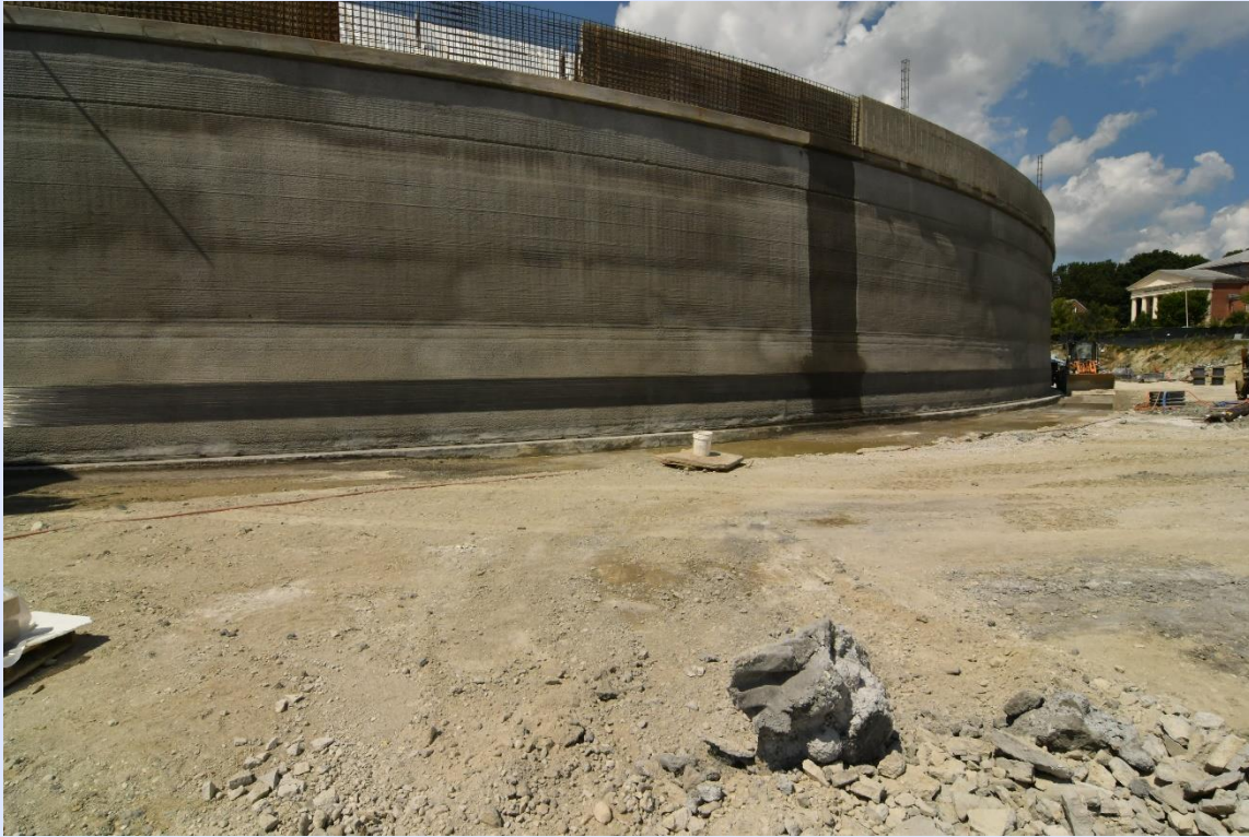
Wire winding at Tank A – 8/26/2022
