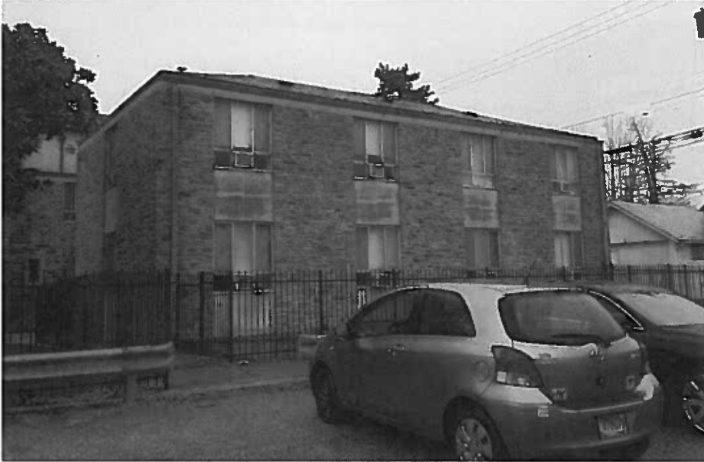
Image 10 – Rear of the 1957 addition.
