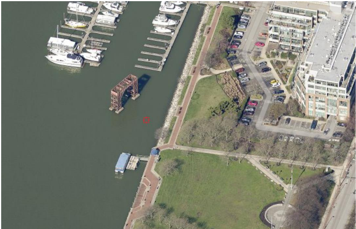
Image 8: Aerial view of Canton Railroad Transfer Bridge from east, Connect Explorer, March 2022
