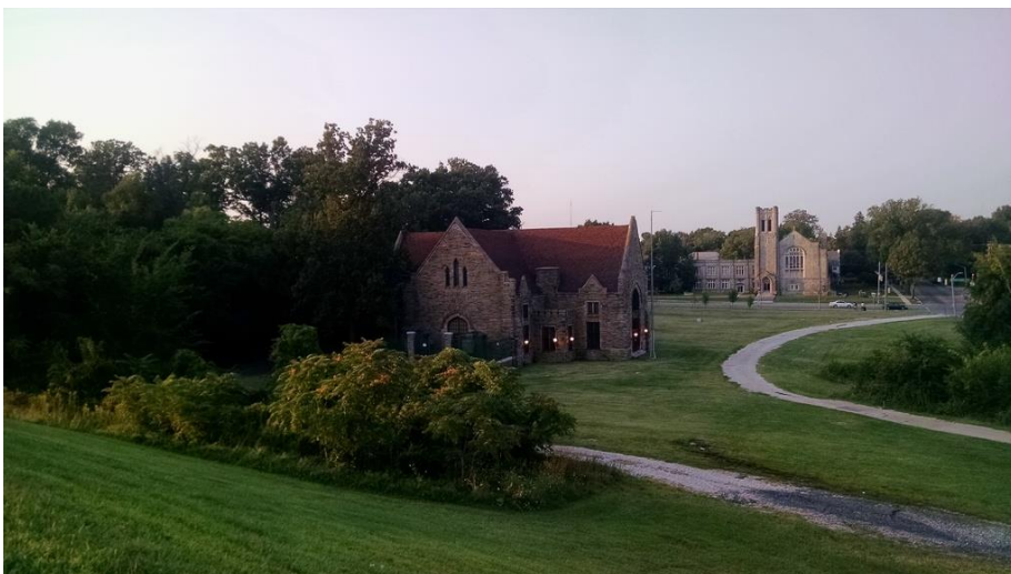
Photo 4: View of Pumping Station from path around Lake Ashburton, looking north, 2015
