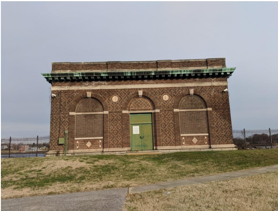
Photo 12: The historic gatehouse at Ashburton Reservoir.
