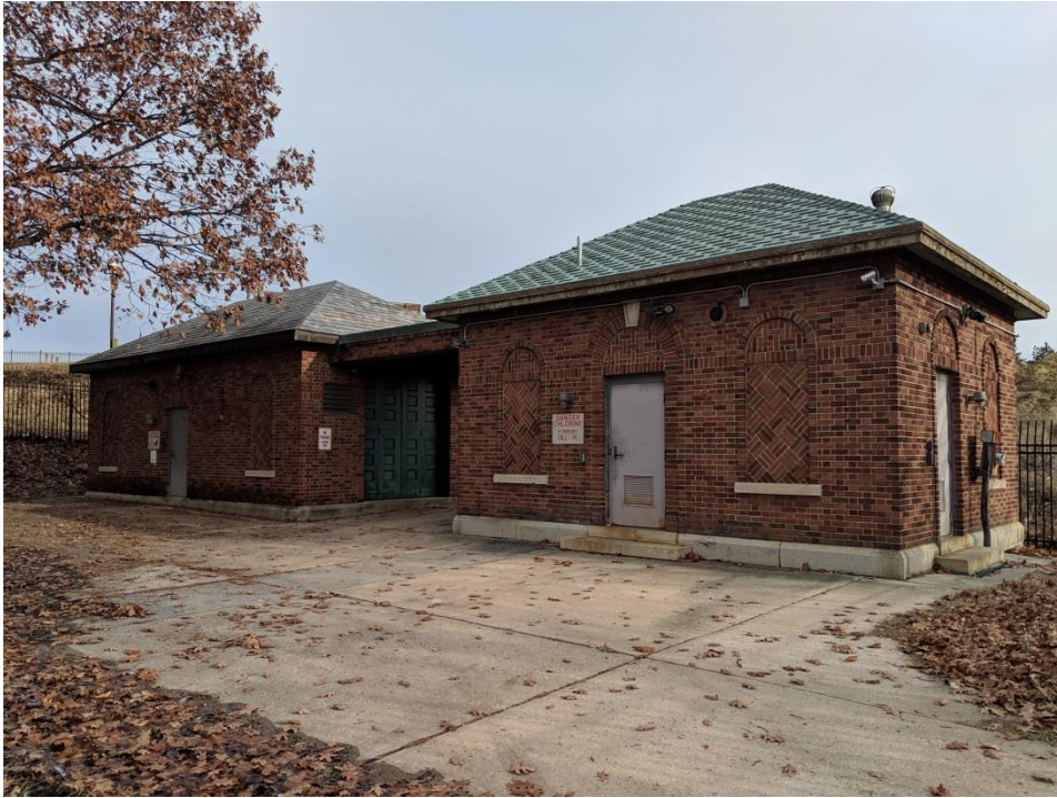
Photo 11: The historic chlorination building.
