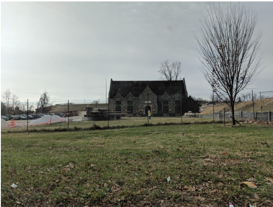
Photo 18: The historic Ashburton Pumping Station, with the reservoir behind it, as viewed from Liberty Heights Ave.
