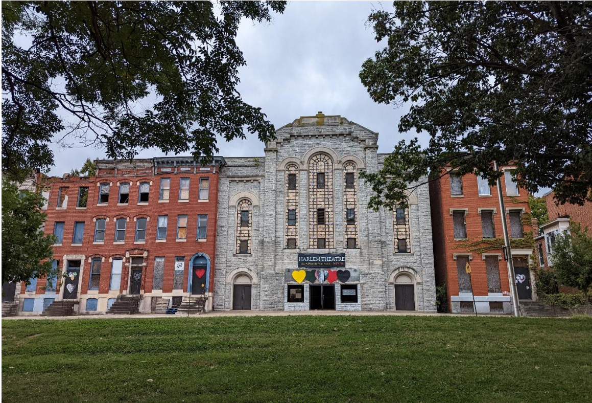
Image 6: Façade of the Harlem Theatre, September 2022
