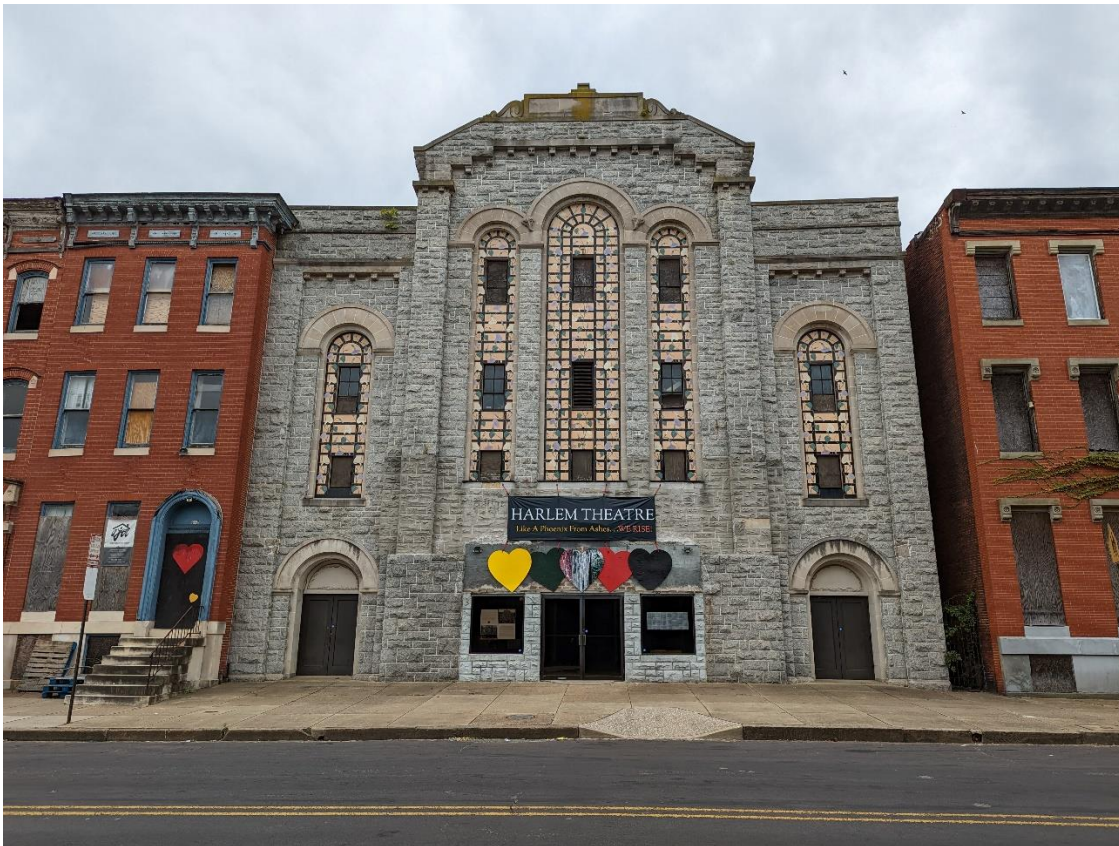
Image 7: Façade of the Harlem Theatre, September 2022
