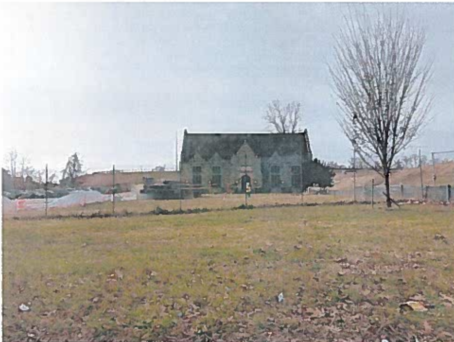
Photo 18: The historic Ashburton Pumping Station, with the reservoir behind it, as viewed from Liberty Heights Ave.
