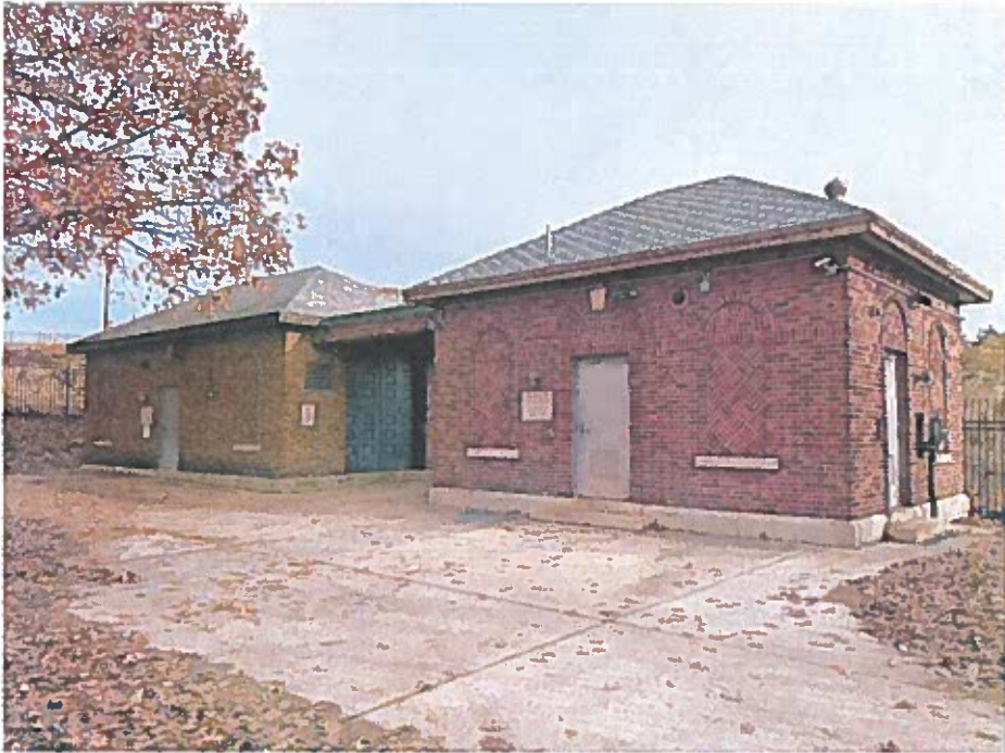
Photo 11: The historic chlorination building.
