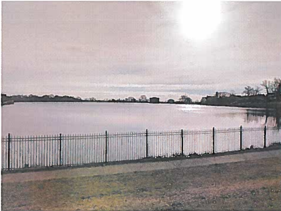
Photo 15: A view of the reservoir looking southeast, with the gatehouse and Baltimore skyline in the distance, and the reservoir fencing and walking path in the foreground.
