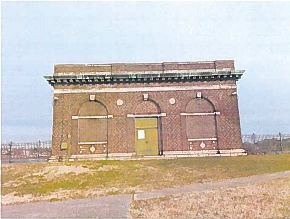
Photo 12: The historic gatehouse at Ashburton Reservoir.
