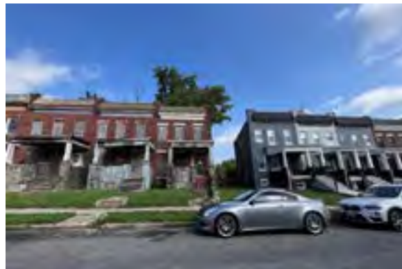
Vacant and renovated houses in Greenspring.
