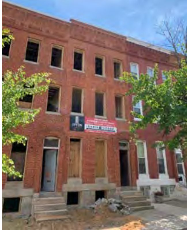
Renovation underway in Upton.
