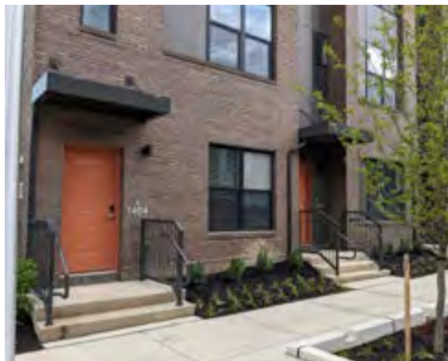
Phase 1 of Perkins completed spring 2024.
