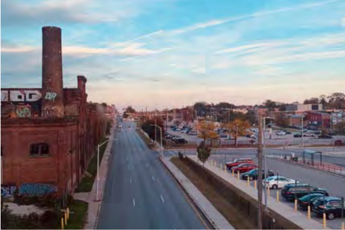
The American Ice Building adjacent to the West Baltimore MARC Station has been the subject of TOD proposals in past years.
