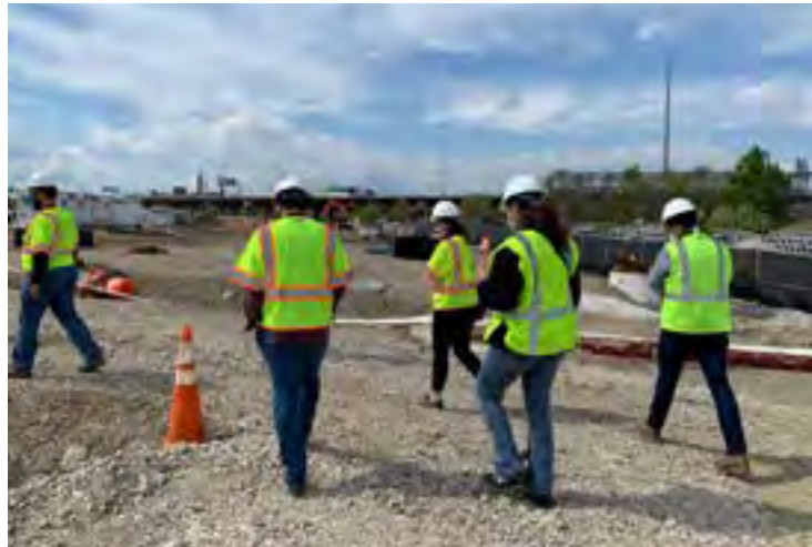
A construction site in South Baltimore.
