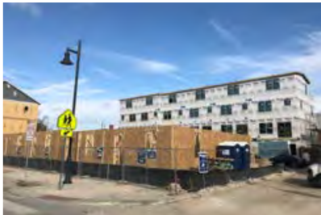
Construction of new residential housing.
