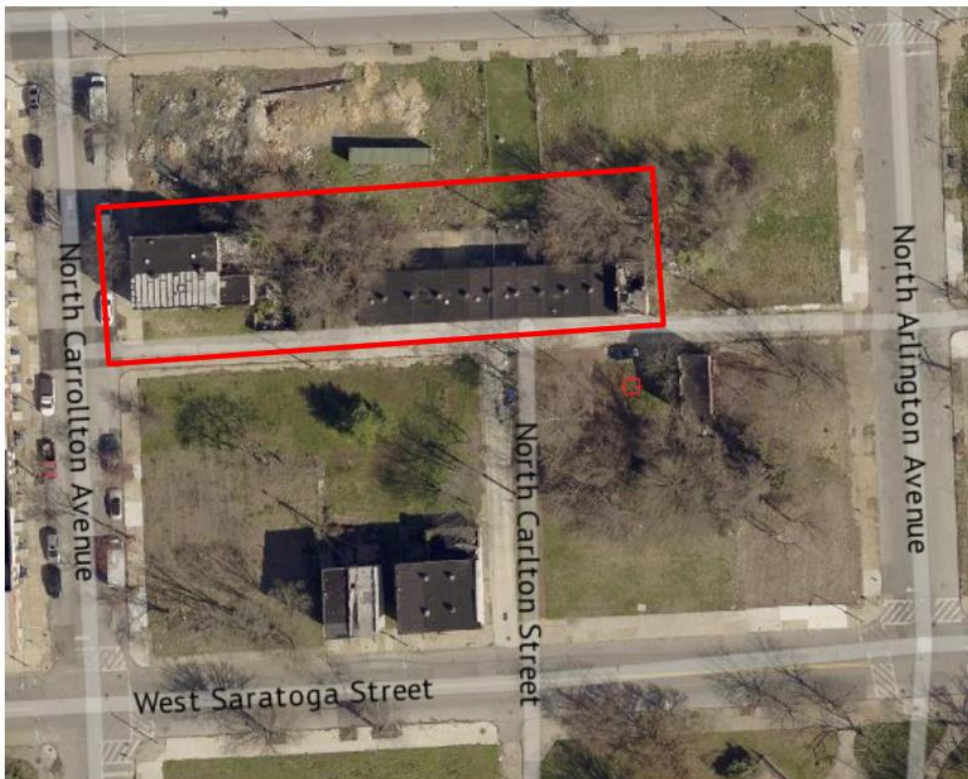
Aerial View of the Proposed Sarah Ann Street Historic District (outlined in red). Connect Explore, April 2022.
