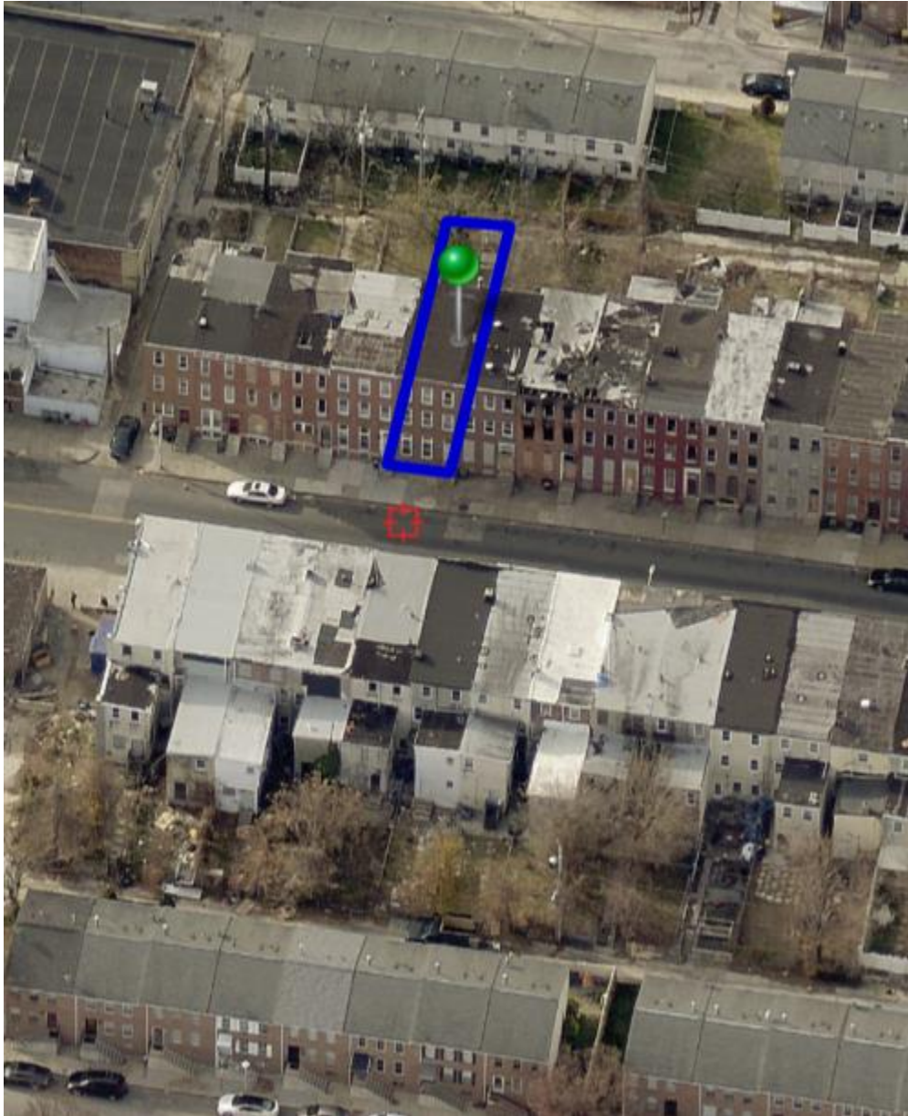
Image 1: 2019 Aerial Photo of property, view from East. (Eagleview)
