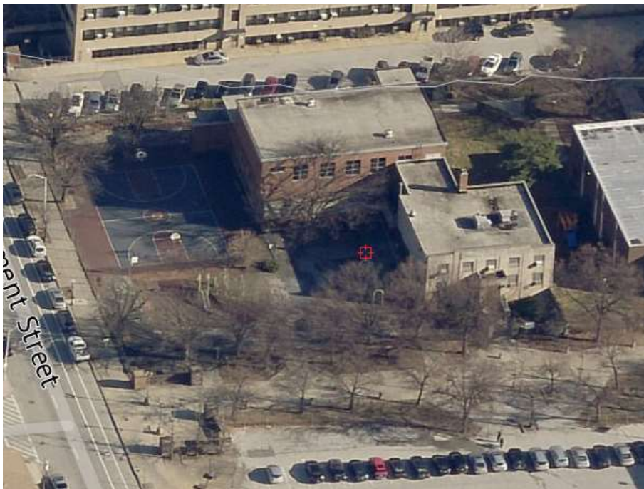
Image 1— Aerial view of site, view from west.
