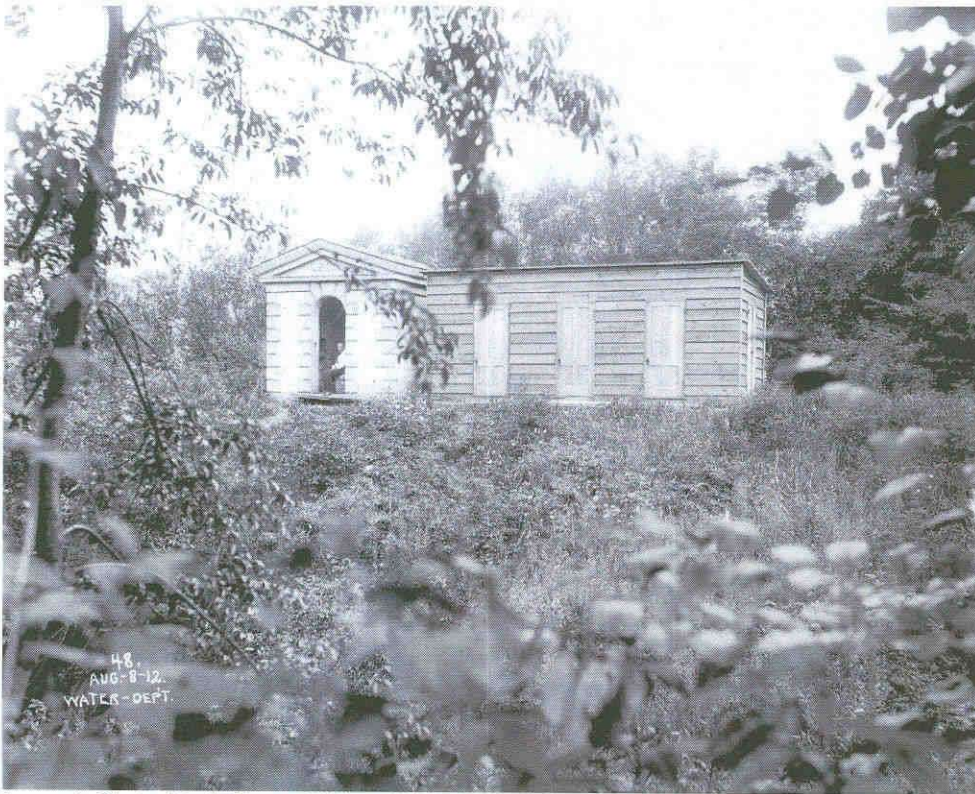
Image 4: Photo titled "Harper's Waste Weir - Roland Supply," depicting the Cross Keys Valve House on August 8, 1912. The purpose of the wooden building is unknown, but may have been used for storage. Courtesy of Ronald Parks, Baltimore City Water Department.
