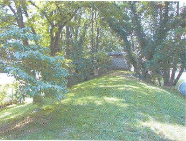
View of the Valve House from the north.
