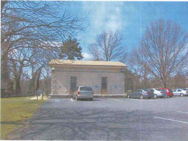
Today, the Hampden Reservoir Gatehouse is used by the SPCA as a Spay and Neuter Clinic.
