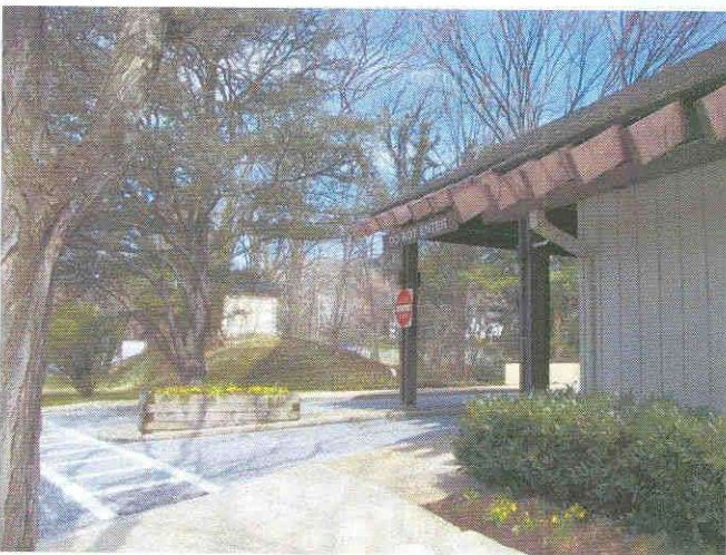
View of Valve House from the south. The building in the foreground is the gate house for the Cross Keys community.
