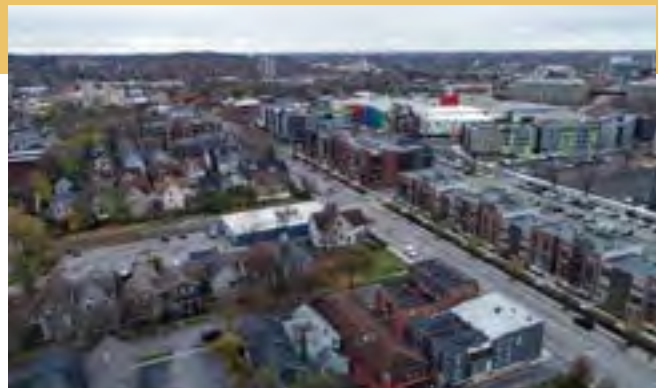
New mixed-income housing constructed after the ditch was filled, Rochester Democrat and Chronicle.
