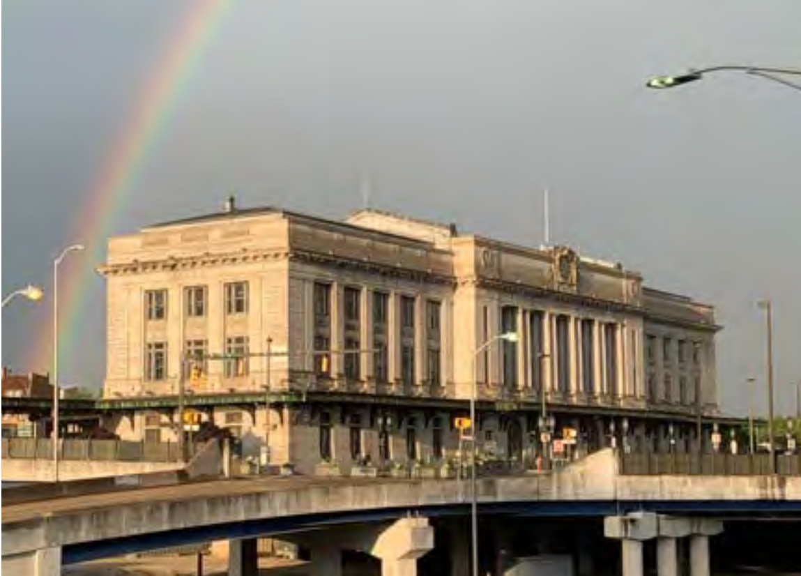
A view of Penn Station from Maryland Avenue.
