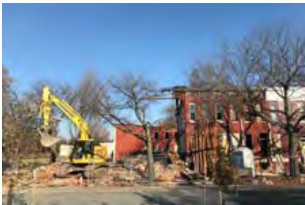
Demolition/deconstruction of vacant rowhouses, 1100 block of E. Hoffman St.
