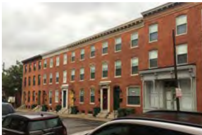
Rehabilitated rowhomes that received the CHAP Tax Credit at 1200 block of Gay Street.
