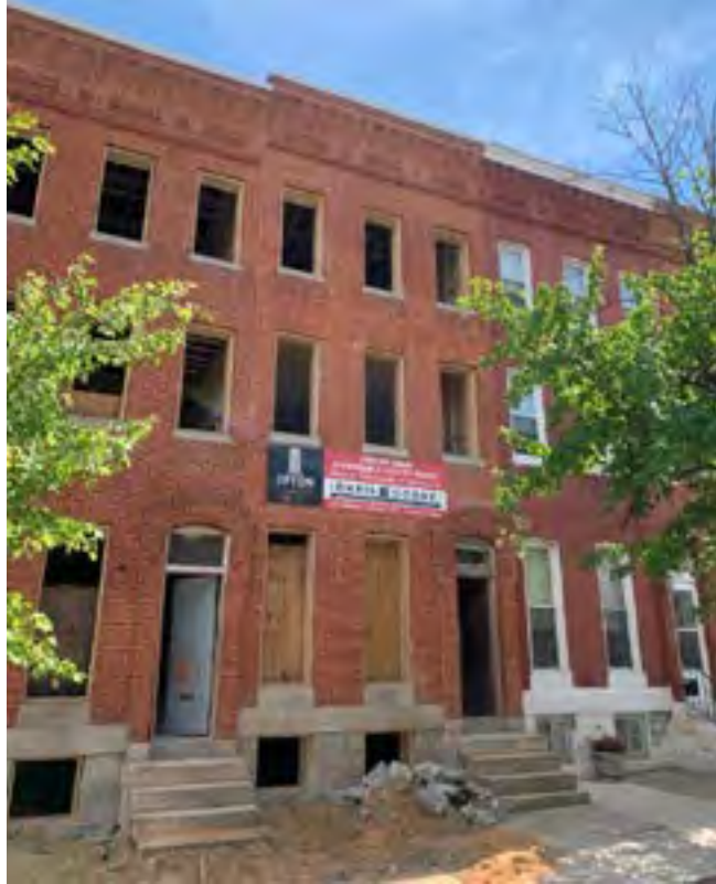
Renovation underway in Upton.
