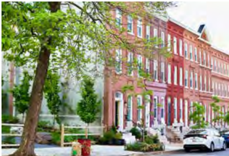
Renovated Homes on Edmondson Avenue.
