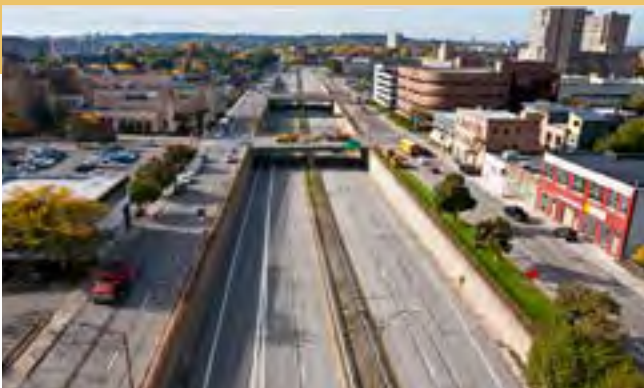
Rochester Inner Loop East, before demolition, Reconnecting Rochester.
