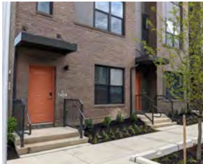
Phase 1 of Perkins completed spring 2024.
