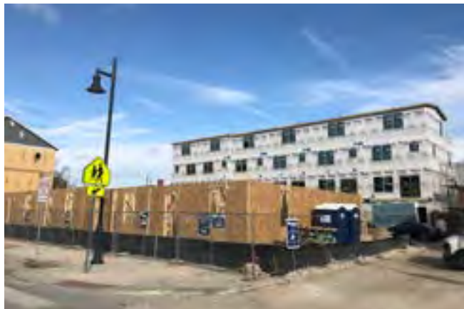
Construction of new residential housing.
