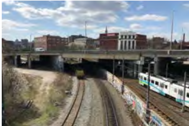
MTA Light RailLink under Interstate 83.
